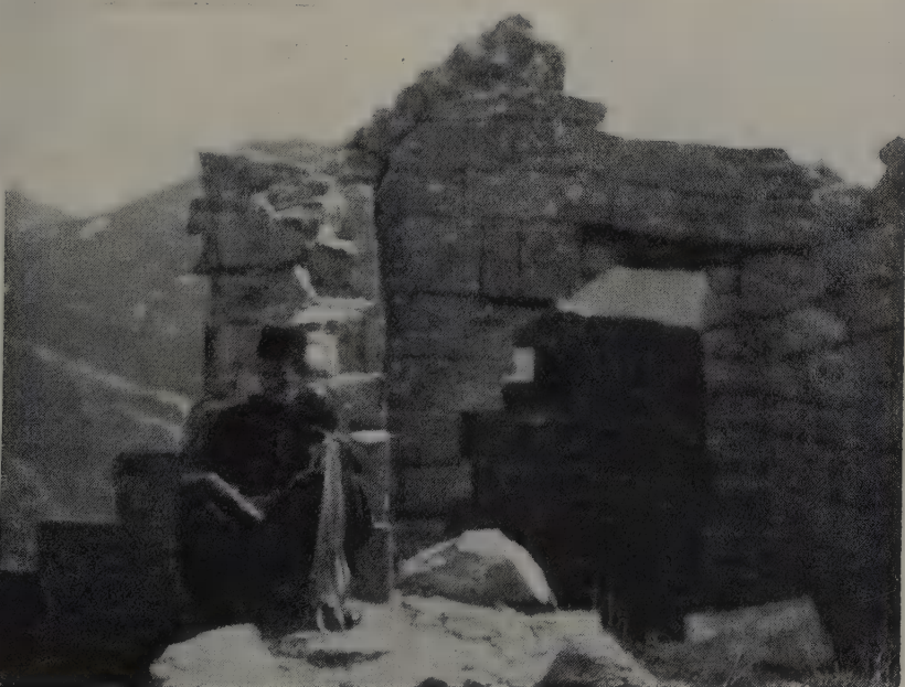
FIG. 119.—No. 31, upper storey of narthex, looking S.
